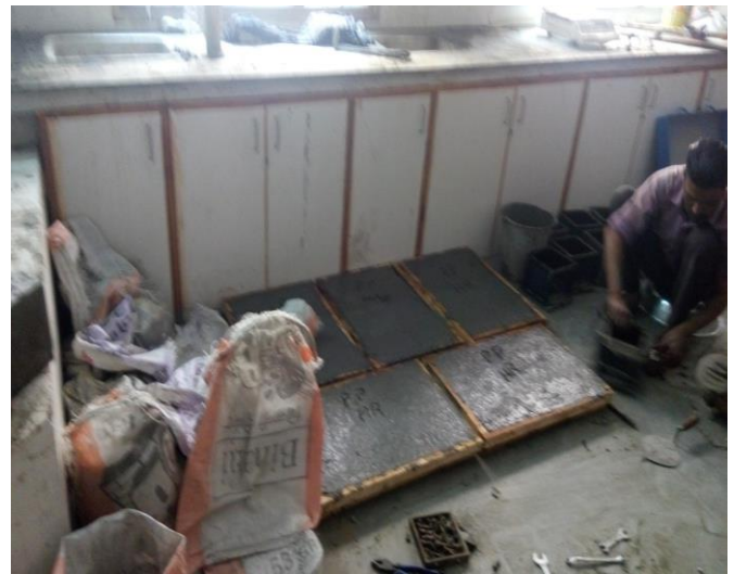
Figure 5: Formwork for SFRC walls
