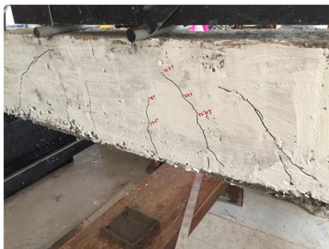
Figure 3. Testing of Control beam
