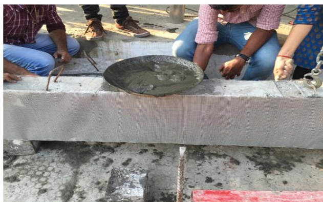
Figure 4. Installation of FRCM
