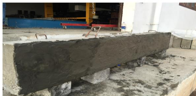
Figure 5. Beams wrapped with 1ply FRCM
