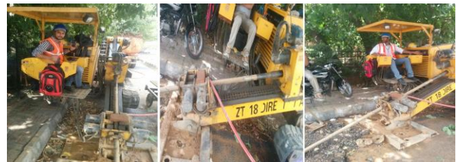
Figure 6: Pipe Ramming In V and A Mesum
