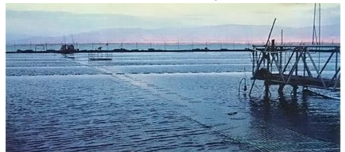
Figure 3: Bet Ha Arava Solar pond power station in the Dead Sea Israel (Ormat, 2002).
