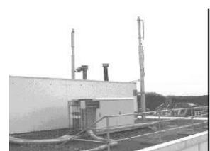
**Figure 2 :** A base station; right: two of the three masts with an antenna at the top; foreground: the equipment cabinet; left: Base station tower with antennas.
