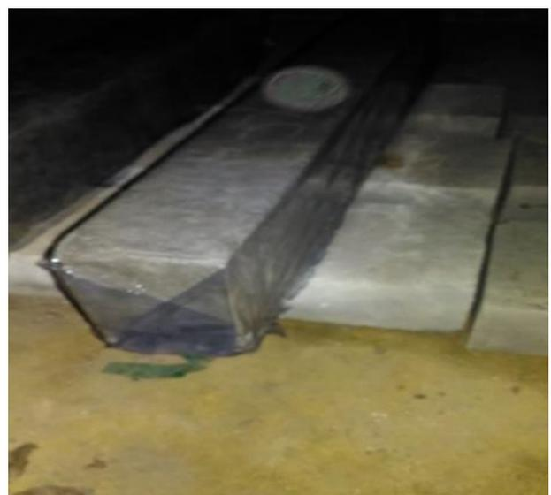
Figure 1. Wrapping Curing
