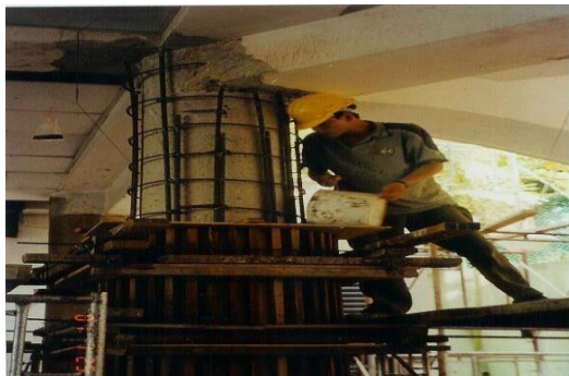
Figure 1 Reinforced concrete jacketing
