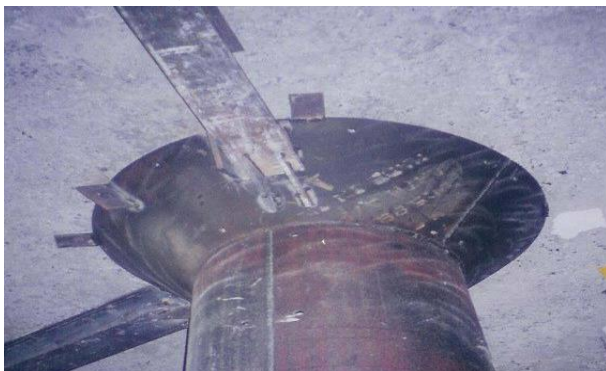
Figure 2 Retrofitting by Steel plate bonding
