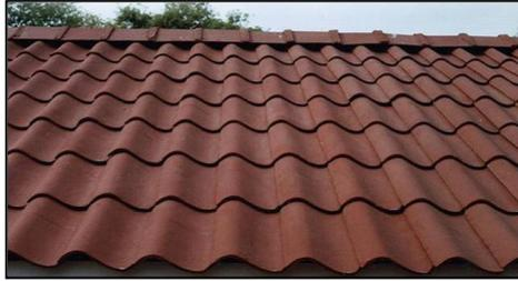
Figure 10. Micro concrete roofing tiles
