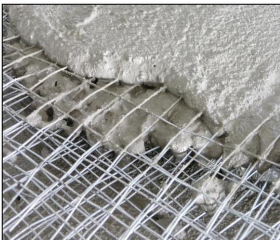
**Figure 2.** Ferro cement and various precast components
