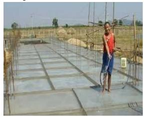
After 24 hour of casting and curing by water were started. It was maintained for 28 days to find strength.
