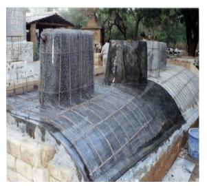
After the surface preparation the material is carried out for the casting. In the casting the different wire mesh layers are used for the better result. First of all the surface is prepared with mortar paste as a thickness then wire mesh is properly laid on mortar. And after above that wire mesh again mortar paste is laid. Is continue as per requirement. And then finally casting is complete.
