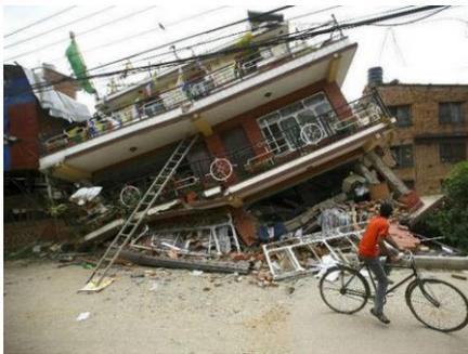
**Figure 1.** Building raised on stilts—with no walls in the ground storey —collapsed.
