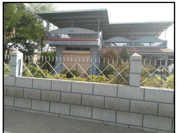
Fig. 8.4 Water Purification Plant
