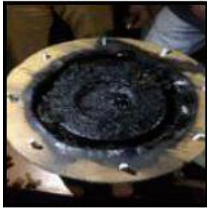
Fig. 7 Removal of moisture
