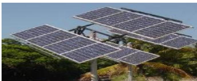
**Figure 4.** Tracking Solar Panel Mount
