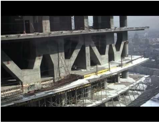
Fig. 5 Concrete Belt truss
