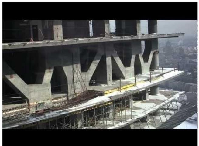
Fig. 5 Concrete Belt truss
