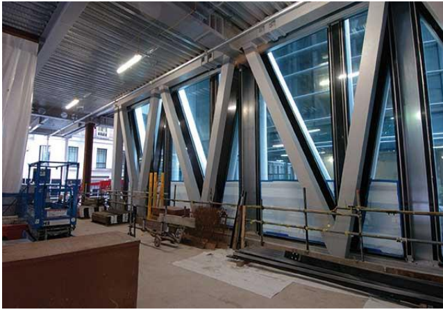
Fig. 4 Steel Belt truss
