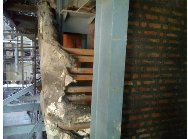
Due to modification of steam drum increases heating area so increases the boiler efficiency. The modification and addition of steam drums tube to increasing boilers efficiency.
