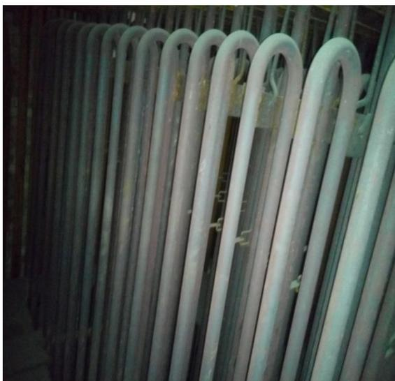
When we add super heaters to increasing the boilers efficiency. The heating area is increases to increasing
