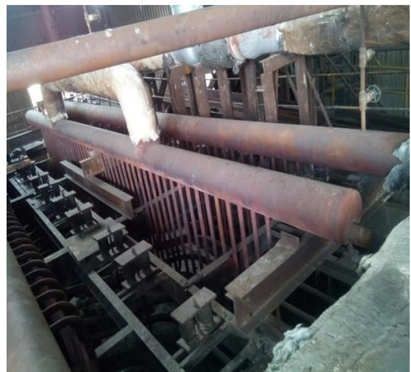
Modifications of steam drums and addition of relief tubes that the bend of tubes from the upper headers to drum .we are the addition of relief tubes to increases the heating surface area. When the increasing the surface heating area to increasing the boiler efficiency .by using this method increases boilers efficiency nearly by 1.78%.
