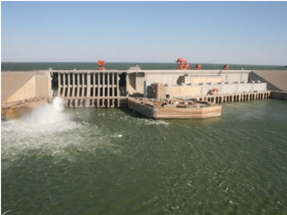
Figure 1. Roseires Concrete Gravity Dam
