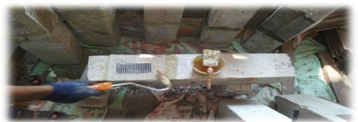
Fig 4: - Wrapping of GFRP inside and around opening
