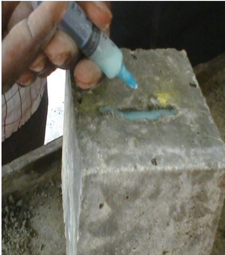
Figure 8. Injecting solution into the crack
