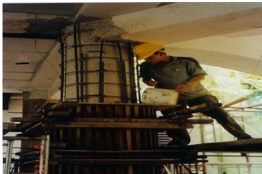
Figure 1 Reinforced concrete jacketing
