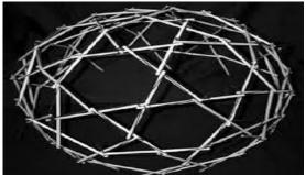
Snelson describes tensegrity as a "class of structure possessing, what may be termed discontinuous compression, continue tension characteristics". Which means the structure will have continuous tension through tout
