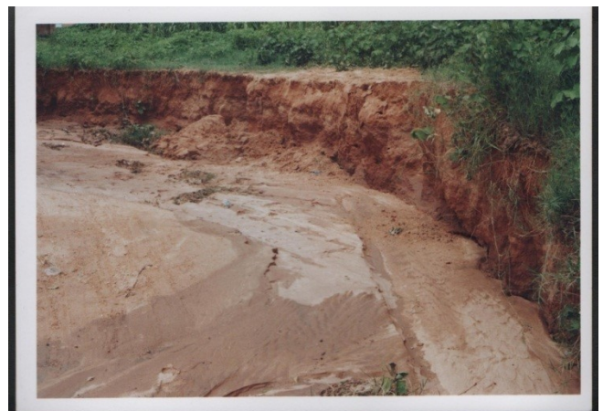
Plate 11. Upstream Area Developed Gully Erosion
