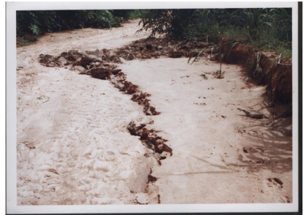
Plate 8. Area where Gabion was used
