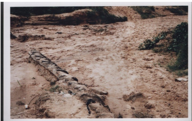
Plate 7. Area where Dyke was Used
