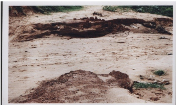
Plate 6. A Eroded Width in The Research Area of Section A
