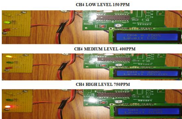
Figure 11. When the CH 4 gas reaches a certain level in drainage channel and display Methane gas and level of gas. If Low level reached then LCD display shows the 150ppm , Medium level reached then LCD display shows 400ppm ,High level reached then LCD display the level 750ppm and corresponding LEDs will glow as per the level of gas present inside the drainage channels.
