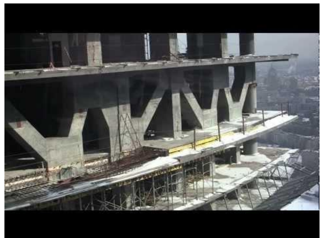
Fig. 5 Concrete Belt truss
