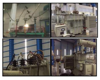
Figure 2: No-load and load test of transformer at industry
