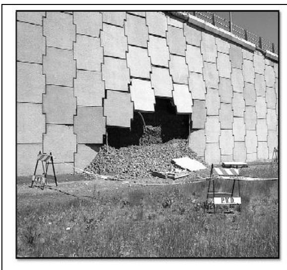
Figure 3. Failure Of Retaining Wall
