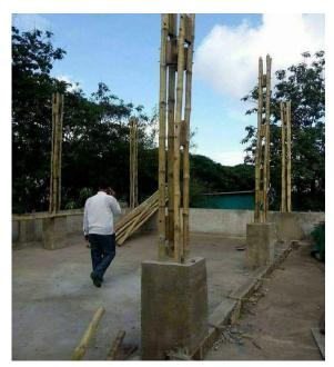
**Figure 2.** Bamboo used to reinforce concrete in beam and columns
