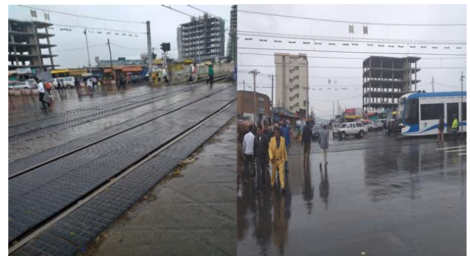
Figure 2. Hazards associated with Rail-Road level crossing at AALRT
