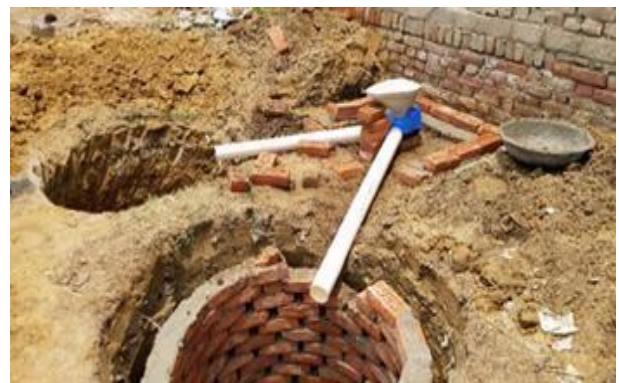
Figure 8 : Eco-san toilet design for village.
