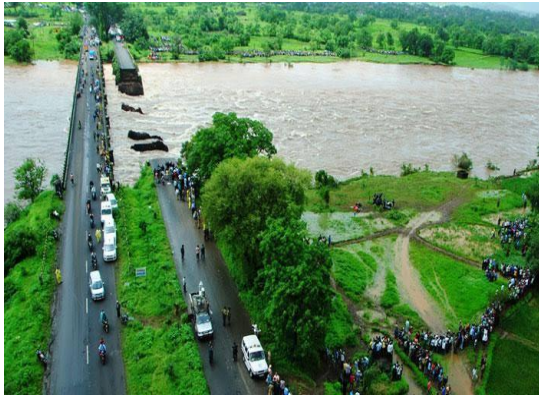
Fig. Bridge collapsed at Satara on the Savitri river
