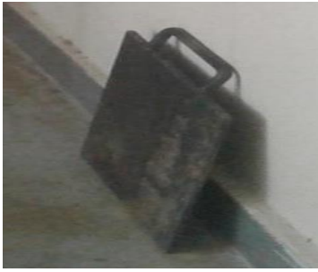
Fig.8 Fabricated opening and closing panel
