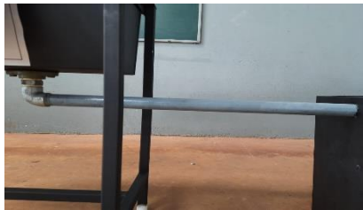
Fig. (3) Connecting Pipe
