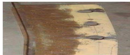
Fig. 4.2 Partial net section ruptures, with large eccentricity
