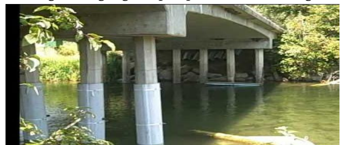
Figure 17. Actual results of using enhanced prefabricated FRP panels
