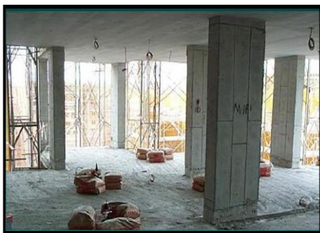
Figure 1.1 : Slabs with columns
