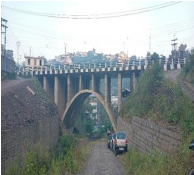
Plate 5: The newly constructed bridge along the river where the old road has been abandoned
