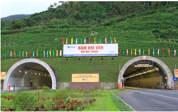
Fig. 1. Hai Van tunnel
