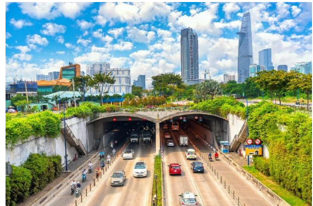
Fig. 3. Tunnel crossing the Saigon River
