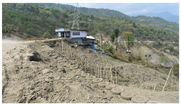
Figure 4: Indigenous treatment of landslide by bamboo hammering downslope of NH-29
