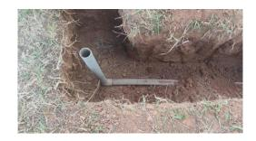
The outlet pipe which is 2m long horizontally and uses an L bend to protrude vertically up to connect the motor. From the whistle 38mm.
