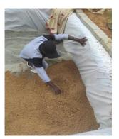
The fine aggregates are used with a size of 2 mm to 4.75 mm. Before spreading fine aggregates, the aggregates
