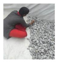
The coarse aggregates are used with a size of 8 mm to 40 mm. Before coarse aggregates are spread, the aggregates are cleaned and dried. After drying, the aggregates are distributed on top of the non-seeping layer.
