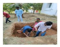
Excavation of wet land for the suitable dimensions of 200cm (length) 300cm (width) on the earth's surface. And a depth of 2.7 m at the level upstream and 2.9 m at the level downstream follows the maintenance of a slope of  $20^{0}$ .
