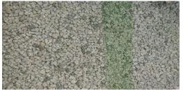
Placement of geotextile on the surface of pre-placed coarse aggregate. The geotextile acts as a separator and resists mixing of one layer with the other layer.
