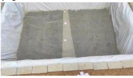
Placement of geotextile on surface of upstream coal. The geotextile acts as a separator and resists mixing of one layer with the other layer.
