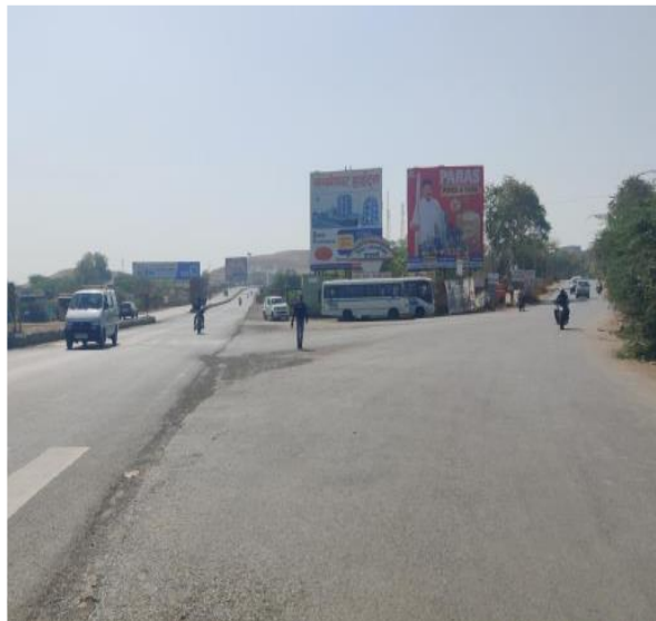
Image: - At Km. 59+600 (Near Shirur Bypass End)
