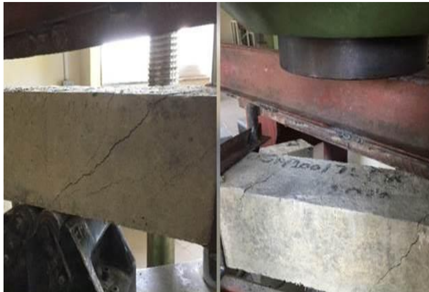
Figure No: 05 Torsional Test failure mode.
