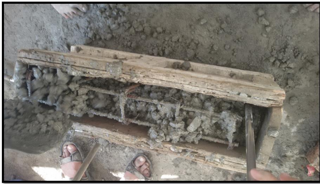
Photo 4. Compaction of beams
