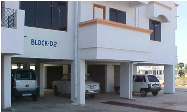
Fig.1 - Open ground Storey of the building
