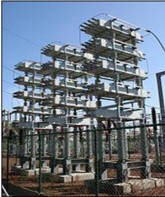
Figure 1. Capacitor banks for PF correction
