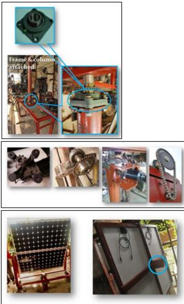
Base of the column is welded and the column being setup
