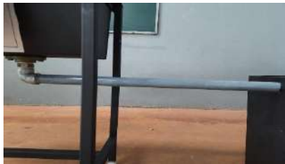
Fig. (3) Connecting Pipe
