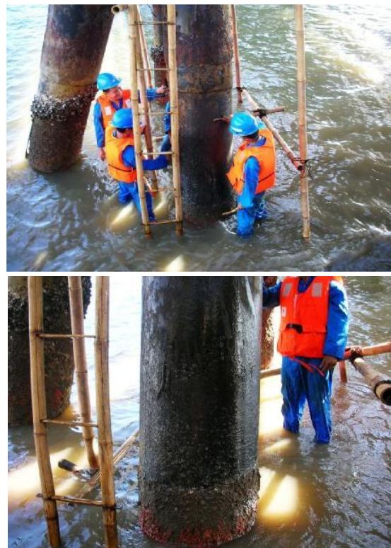
Figure 14. Strengthening the bearing capacity of the pile foundation structure
