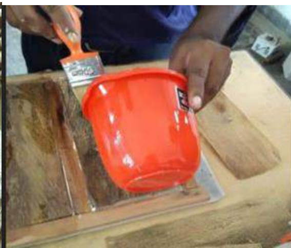
Fig.6 Pouring of resin Mixing
